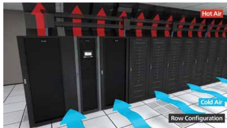
*Innovative thermal management options of front-to-top or front-to-back airflow.*
